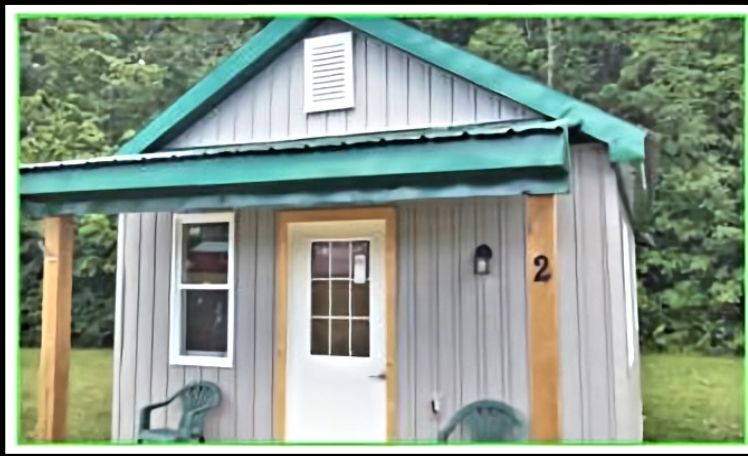
Mill Stream Boys Cabin 2 Completed!
